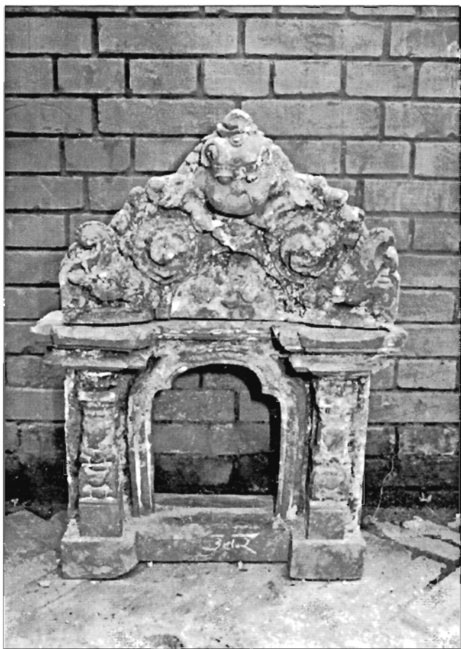
Terracotta before cleaning (Deteriorated by white calcarious material deposition)
