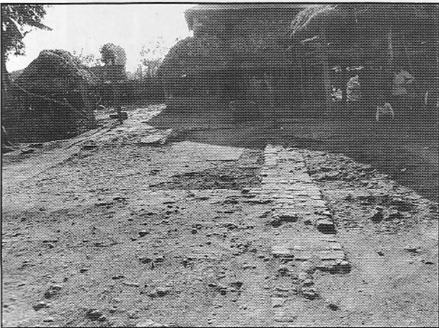
c. Wall structure seen on the surface
