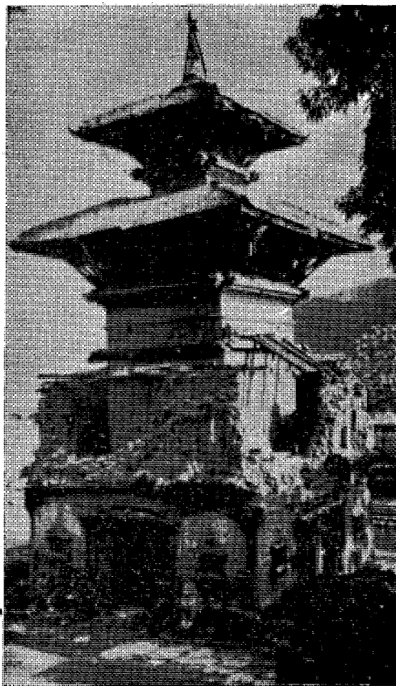
(A) Brahmayani Temple before restoration
