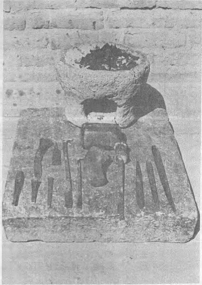
Sculpting tools and brazier (right: horn tools; left: metal tools). (page 42)
