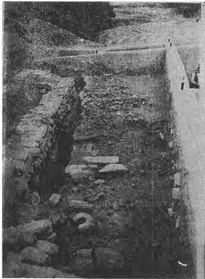
Plate IV: Flooring and Walls, Looking North
