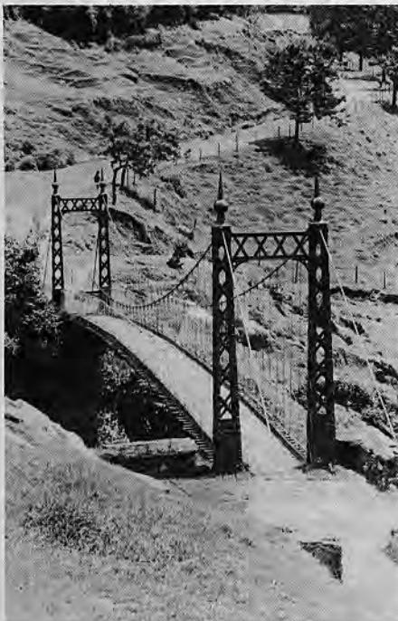
Chandra Sumshere's Scottish Bridge.
