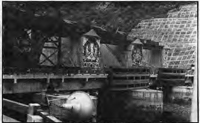
The dam across the Wang Chhu at Chukha in southwest Bhutan.
