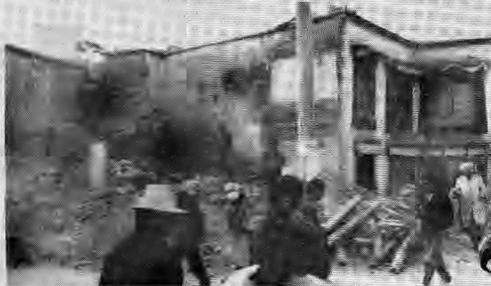
A Barkhor section being demolished in early September.
