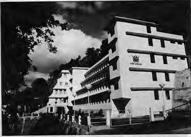
The Department of Power, Gangtok.
