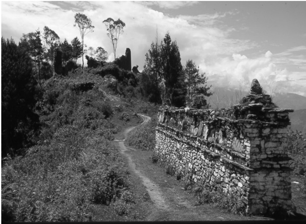
Figure 9: Ruins of Tsenkhar Castle, Photo by John Ardussi
