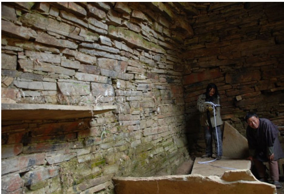
Figure 8: Inside the Bangtsho Underground Fortress; Photography by Kuenga Wangmo, 2014.
