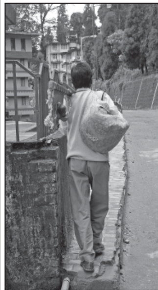
A section of the newly constructed 'foot' path (literally) near the Nirman Bhawan. a Midweek photo.
