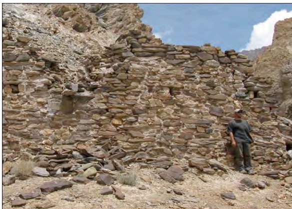
Fig. 42: Mixed-stones masonry. Wall of building A, castle of Tinley Katpa. [credits: Devers 2009]
