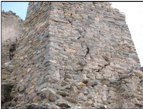
Fig. 41: Multi-colored cobble masonry with timber lacing. Timber lacing is a sign of more modern construction. Tower of Markha, the wall is about 2.5 m long. [credits: Devers 2009]
