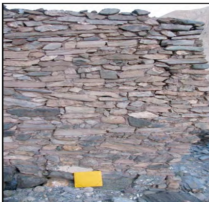
Fig. 44: Masonry with a predominance of schist. This wall is one of those made with red mortar at Hankar. [credits: Devers 2009]
