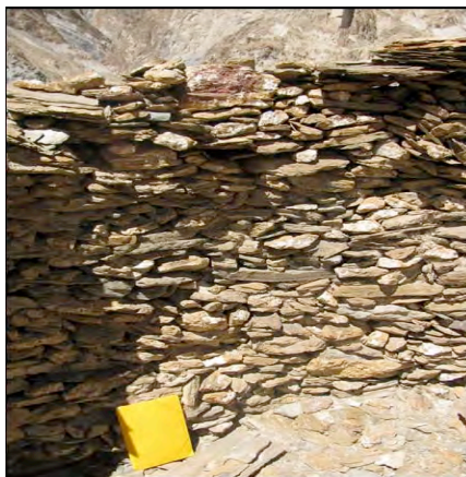
Fig. 43: Masonry with a mix of schist and small stones. The latter are 2 to 3 cm in diameter and are between the slabs of schist. Such stone works have little to no mortar. The yellow folder is 24 x 31 cm. Wall of the circular room downhill of tower C, Pentse. [credits: Devers 2009]
