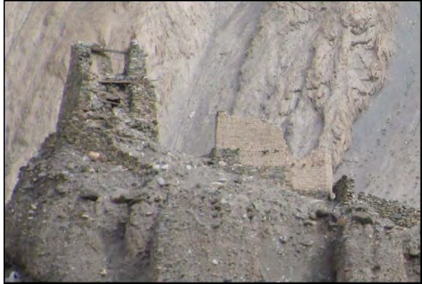
Fig. 22: Markha: tower of the northern crag (left, mud-mortared stones) and possible grainhouse (right, mudbricks: 40x20x10 cm) viewed from the west. [credits: Devers 2009]
