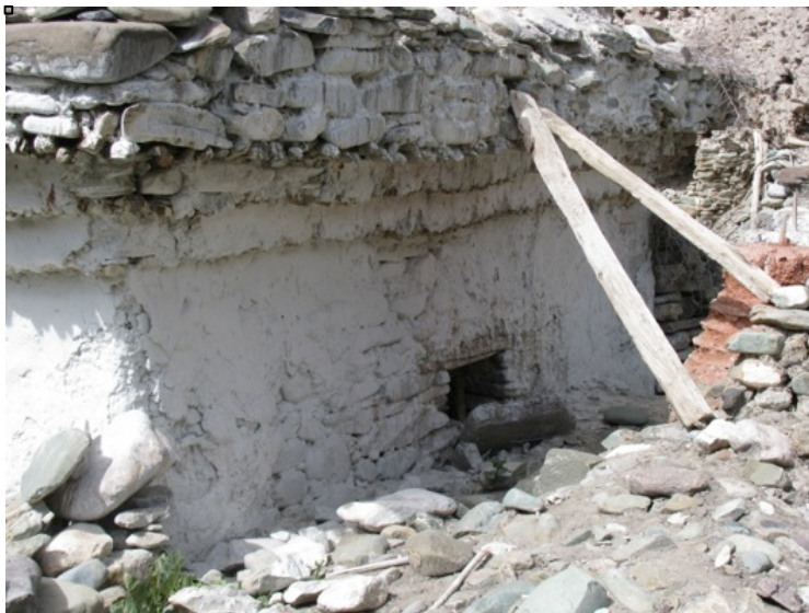
Fig. 3: Half-buried entrance. (Devers 2009).
