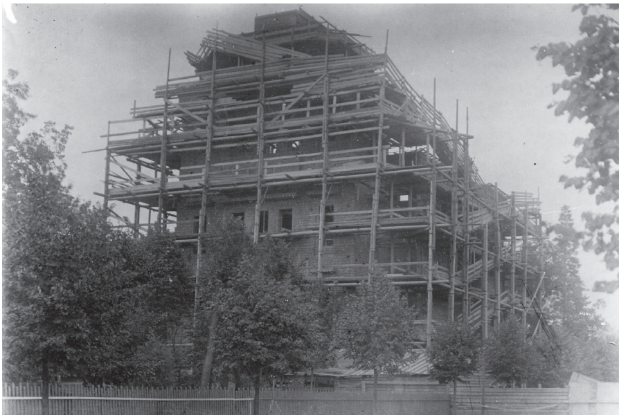
Cracow Construction of the Buddhist temple in St. Petersburg, probably 1909 (see Andreev 2012, p.50). Photo 14626, K III-19, 160, Archive of Science of PAN and PAU.
