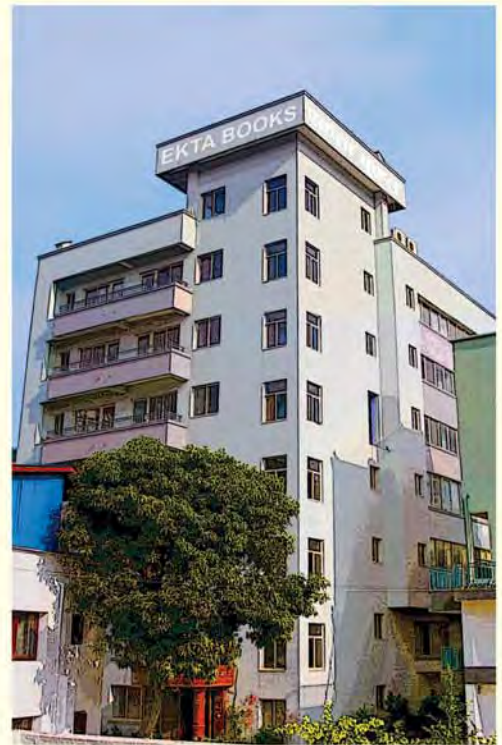
Our Corporate Office Building
