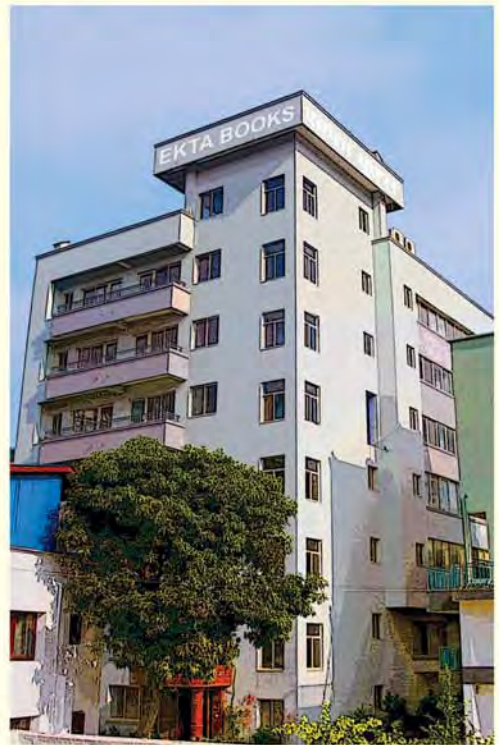
Our Corporate Office Building
