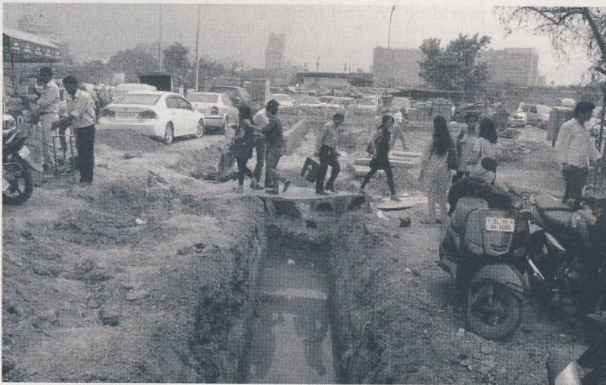
Ground Construction For Common Wealth Games : Work in progress
