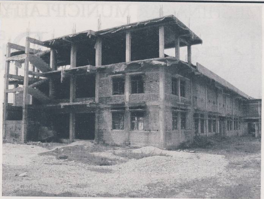
Pending work of Community Building of Kakarvitta: Mismanagement
