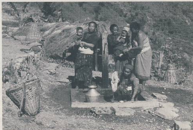
Drinking Water Tap
