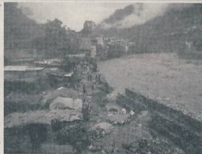
Flood: Curbing Damage 22
