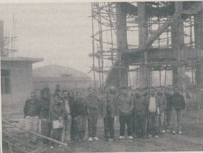
Drinking water project in Meghauli, Chitwan
