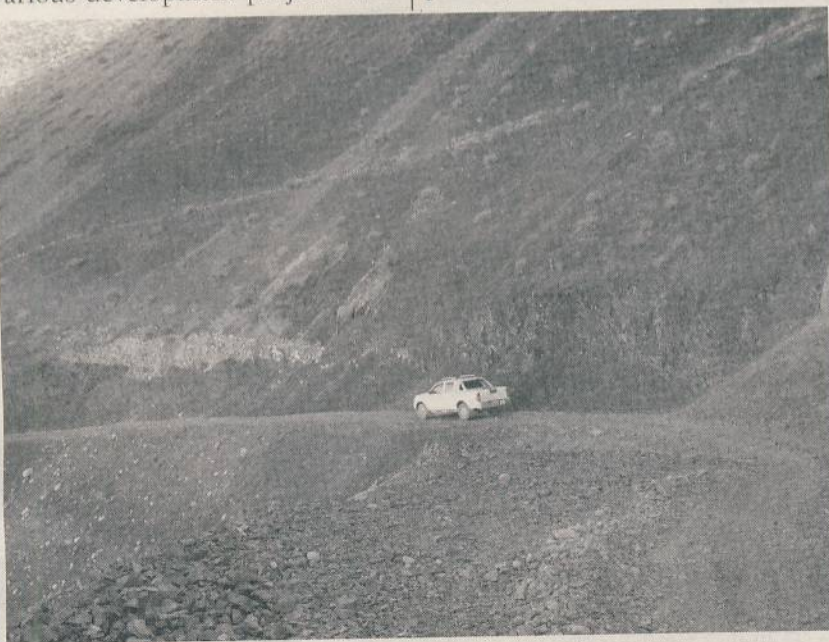
A section of Kagbeni-Samar road
