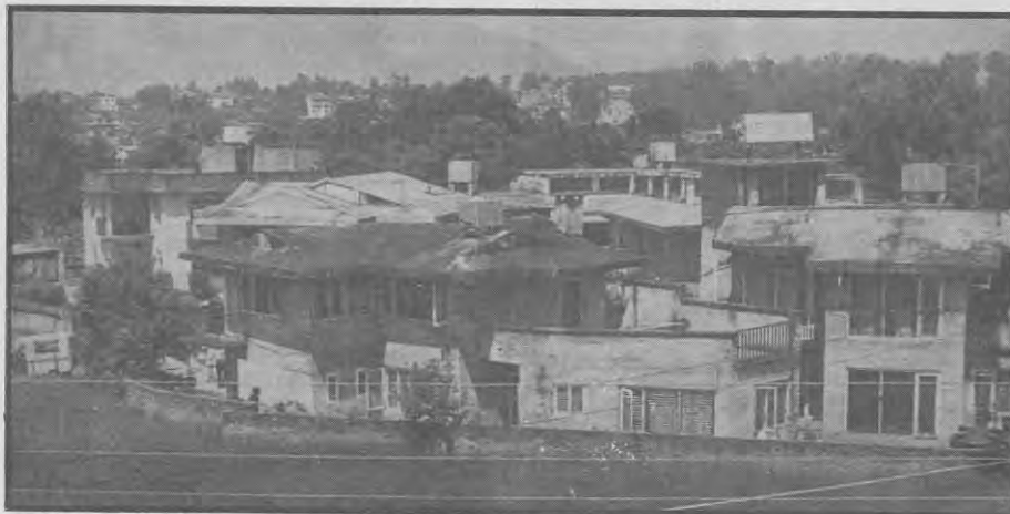
Buildings in Kathmandu : How safe?
