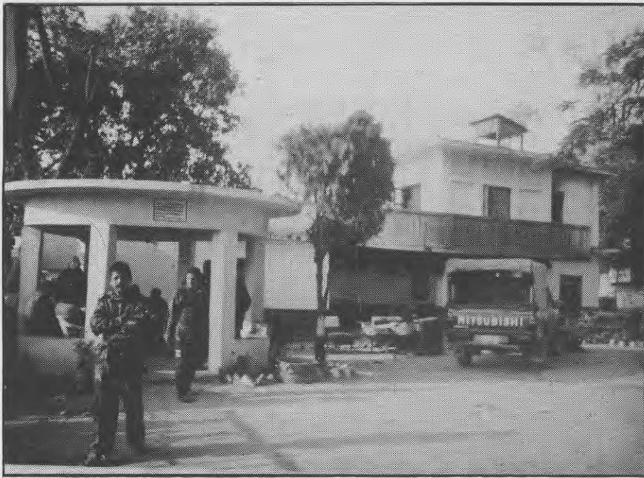
District Police Office in Dang : Failing to protect itself
