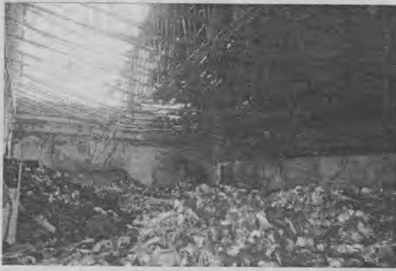
Destruction of a spinning mill: Damage to industries
