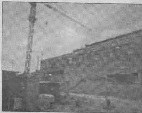
Building Under Construction
