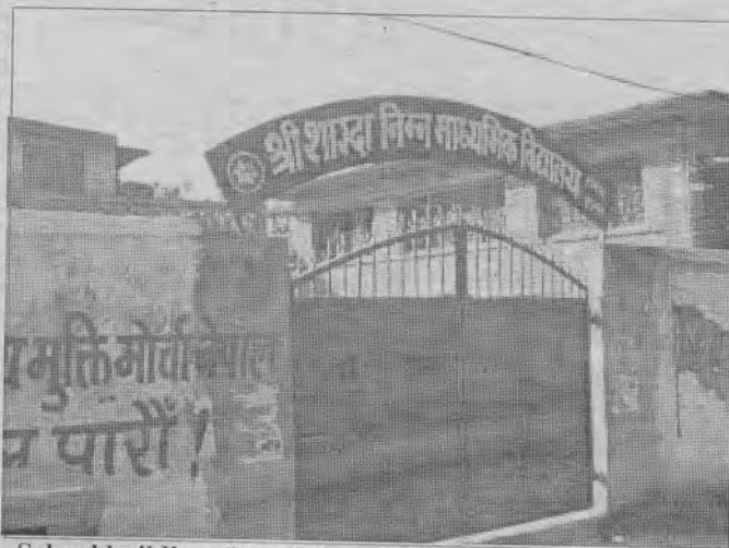
School building: Poor infrastructure
