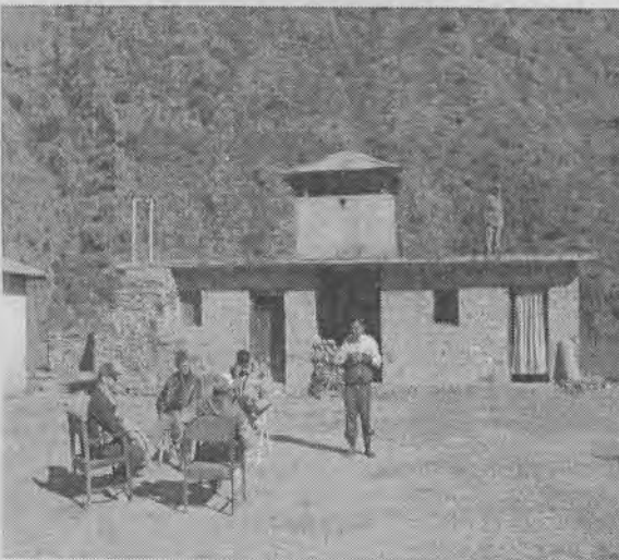
Newly restored police post: Changing scene installation and wires placed in and
