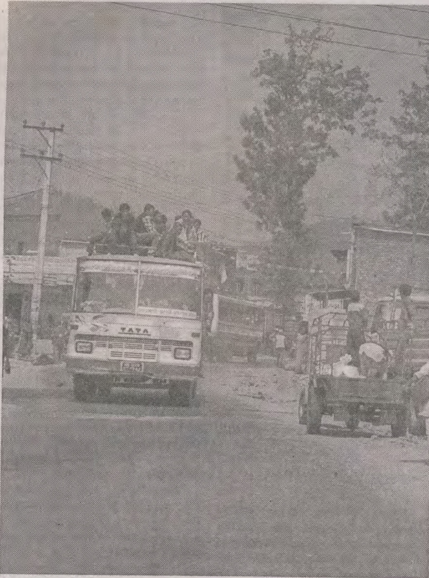
Road Infrastructure: Solid foundation
