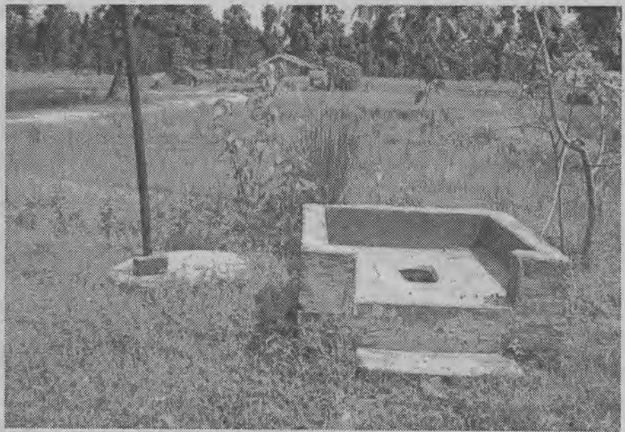
Construction of Latrin : Where money goes ?
