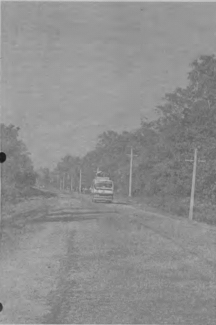
East West Highway in Tikapur : Road under cease
